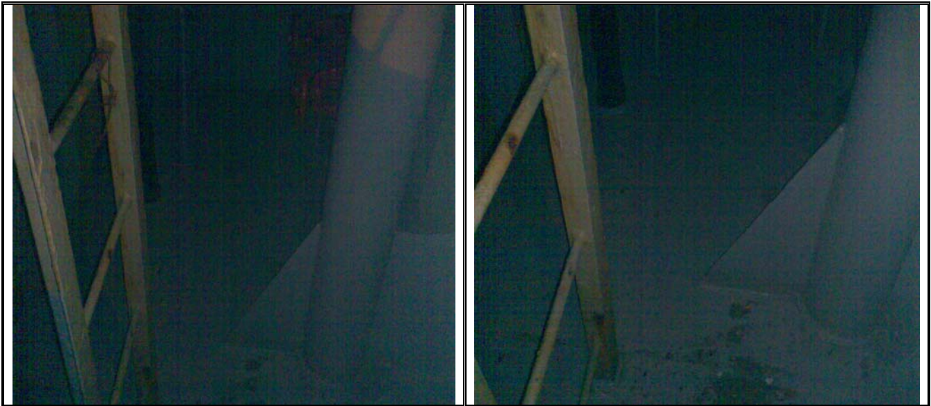
Descaling using Chain Links
